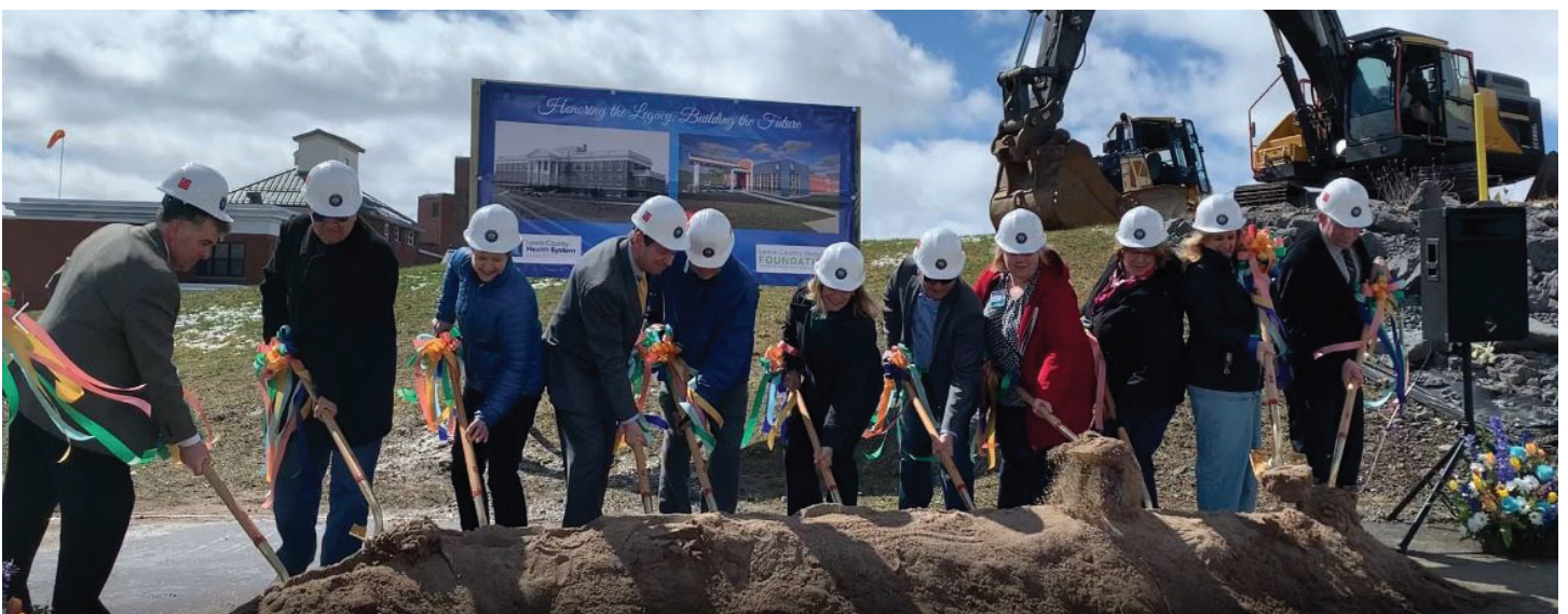
Members of the Lewis County Board of Managers, Lewis County Hospital Foundation, LCHS medical staff and employees participate in the official project groundbreaking.
